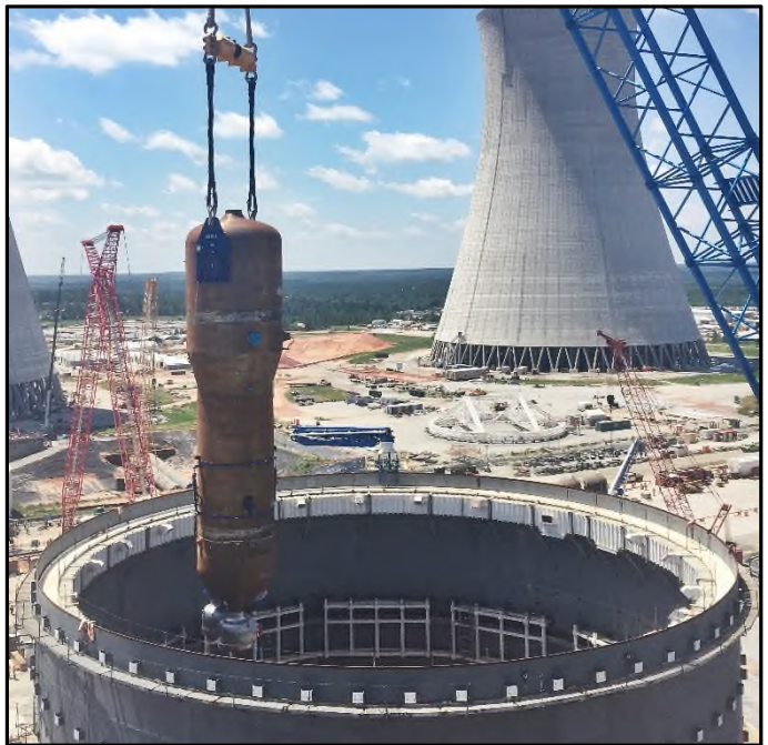
Photo 2 – Setting of Unit 3 Steam Generator
