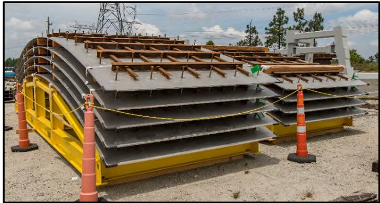
Photo 1 – Unit 3 CB20 PCS Tank Panels
